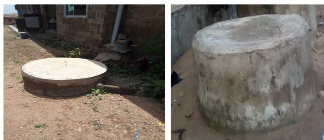
Figure 1 Examples of modified septic tank units within study area.
