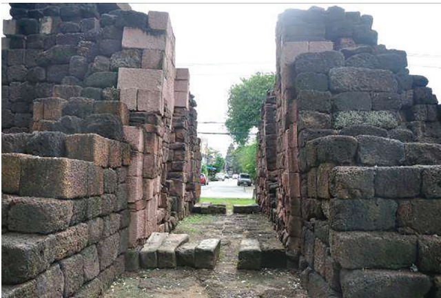
FIGURE 18 Stone jambs of the doors in the West Gate. View from outside the town (author's photo, 2017)
