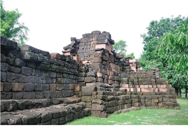
FIGURE 10 View of the North Gate from outside the town (author's photo, 2017)
